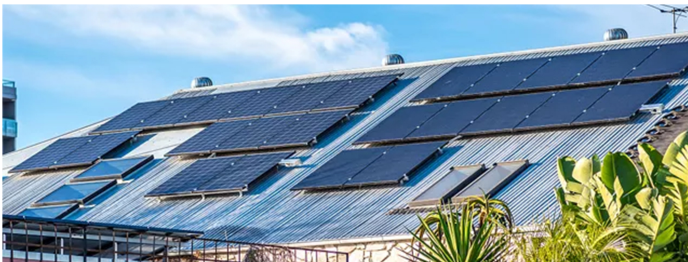
205 MW PV plant in Milan, Italy
