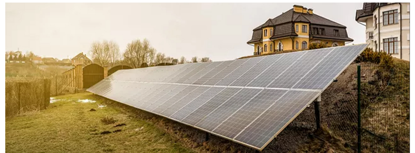
168 MW PV plant in England, UK
