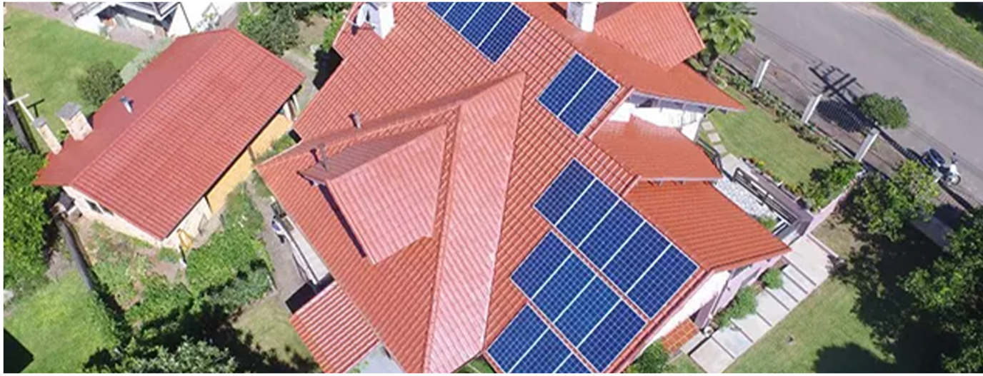
5.9 kWp Sistema FV Birmingham, UK Residence
